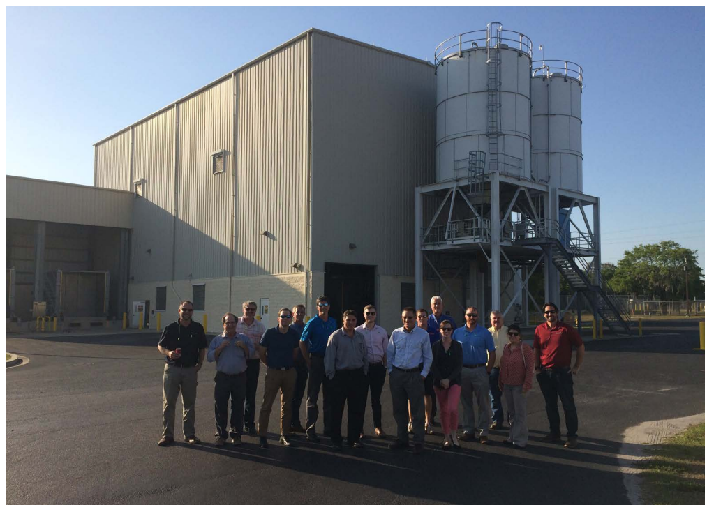
Members in front of Manatee County's Biosolids Dryer Facility
