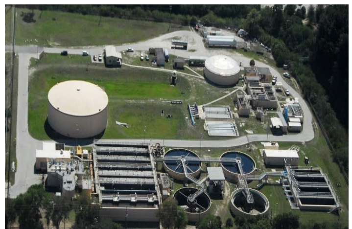
Figure 1: WRRF at Completion of Construction
