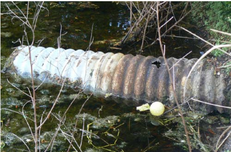
Corrugated Metal Stormwater Pipe in Country Place Subdivision
