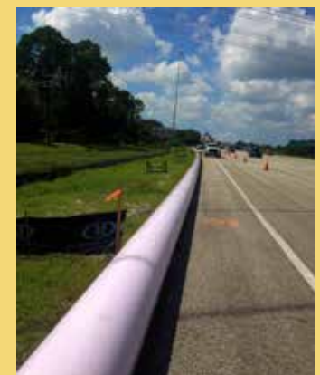
20-inch fusible PVC staged for HDD pullback during construction.
