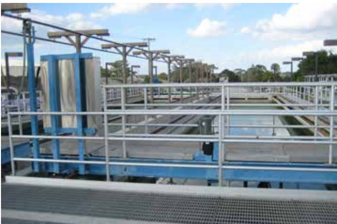
Rehabilitated filters at Manatee Southwest WRF.
