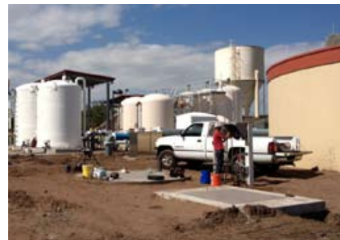
Arcadia Ion Exchange WTP Construction
