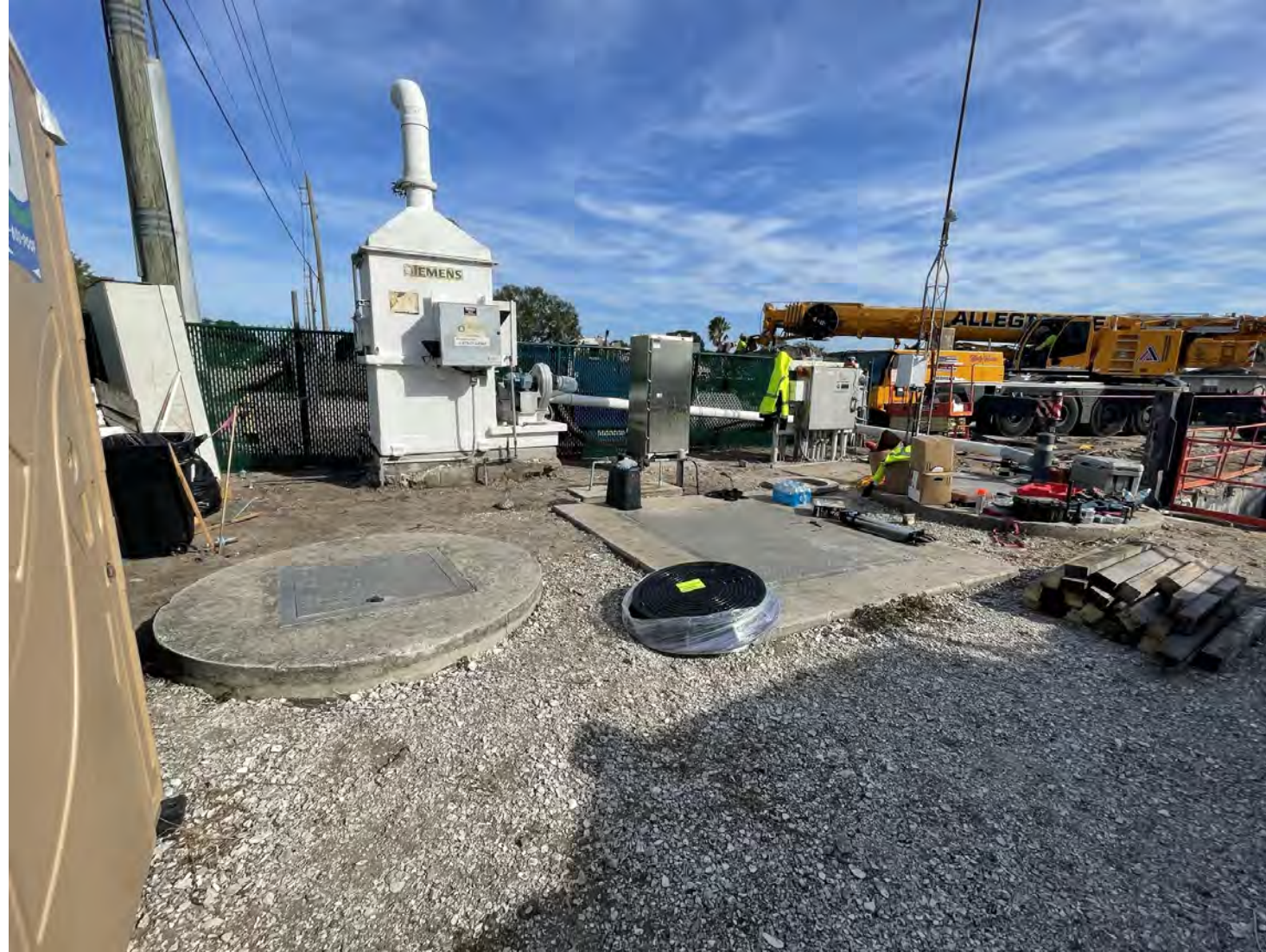
Old Design With Concrete Structures and Odor Control Pulling Air Only From The Wet Well
