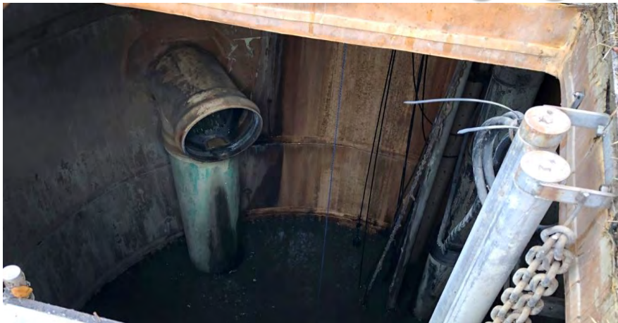
MLS CC6 H2S Before & After Covering Drop Pipe
