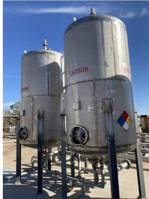
Siloxane Removal Vessels
