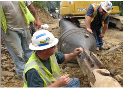
SETUP FOR DIRECTIONAL DRILLING WITH DI
