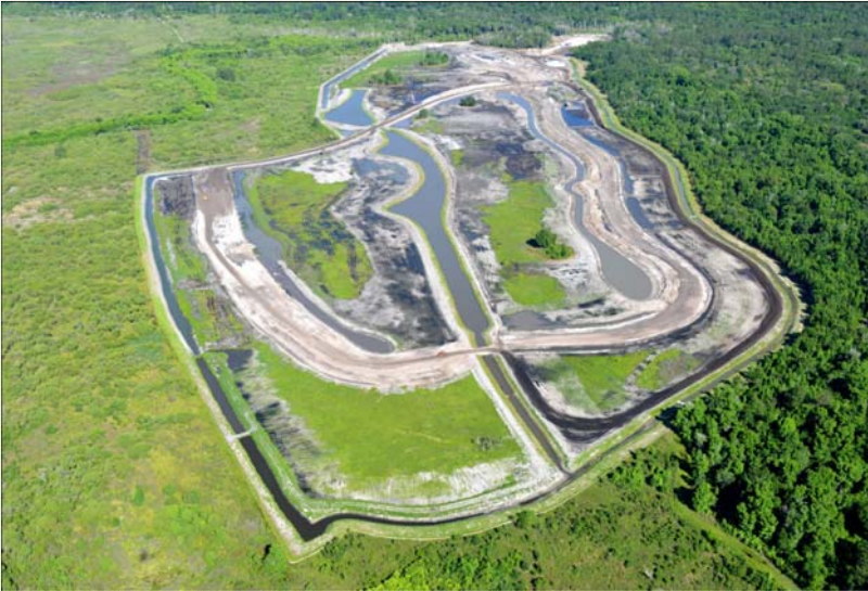
Figure 3 Enhancement Wetland Construction – April 2013
