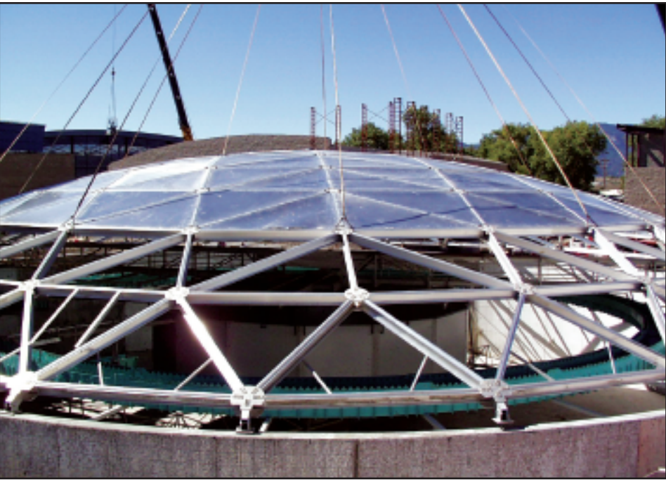
A dome is lowered onto a clarifier during construction. Since the Northern Water Reclamation Facility is surrounded on three sides by residential and commercial areas, addressing residents’ concerns about odors, traffic, and aesthetics was a high priority.
