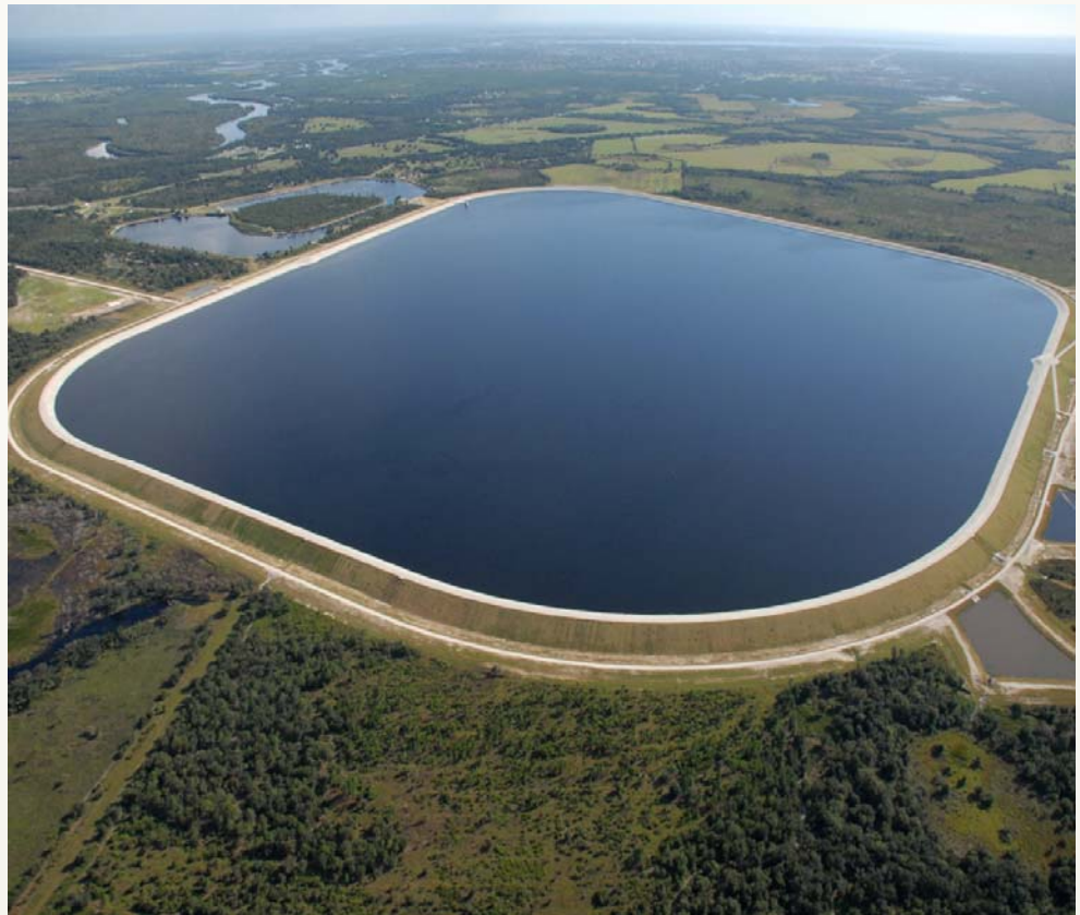
Reservoirs No. 2 (foreground) and No. 1 (middle left) with the Peace River winding its way to Charlotte Harbor (top)
